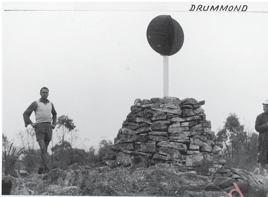
Drummond Trigonometrical Station - Original rock cairn. In this photo the pole and disks have been repaired and the rock repiled.
